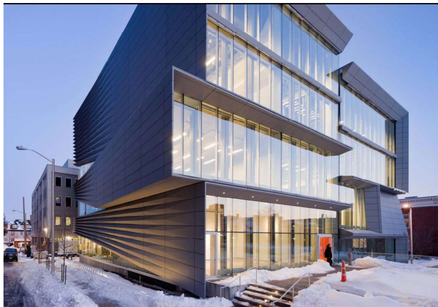
view from north west corner
